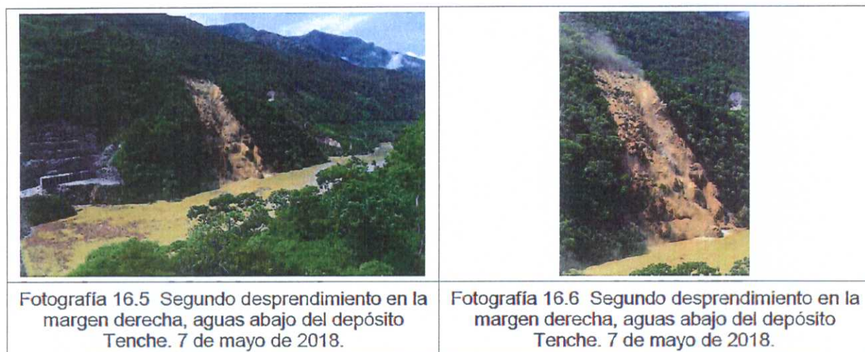
Figure 42. Landslide on the right bank of the river May 7, 2018 219
