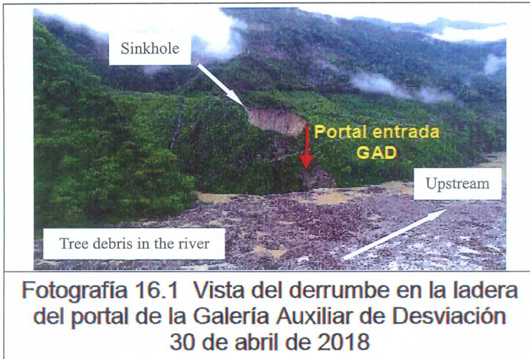
Figure 39. Photograph showing sinkhole and landslide above the ADT on April 30, 2018 212
