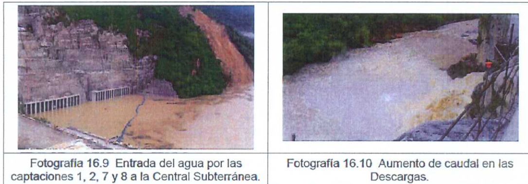
Figure 45. Photographs showing the conditions on May 11, 2018 225
